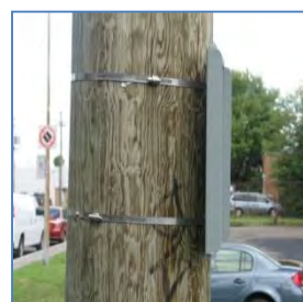
Figure 16, Profile view of pole bracket
